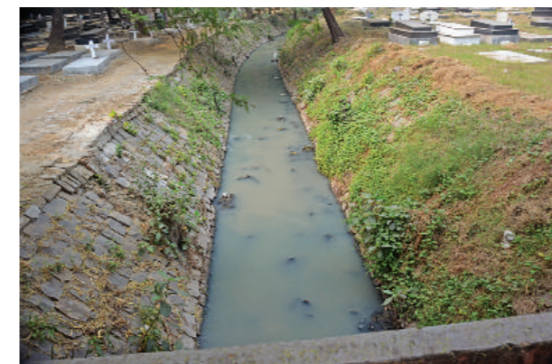
Embankment along the Nullah, Nicholson Cemetery
