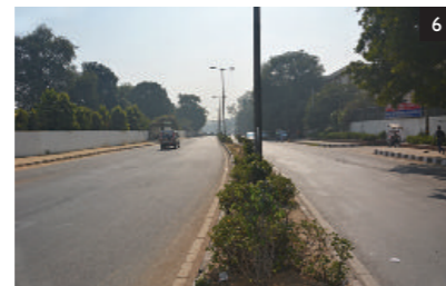
6 Pedestrian walkway along Shamnath Marg
