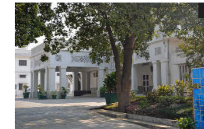
5 Canal Rest House, Shamnath Marg
