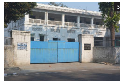
Canal Rest House, Shamnath Marg
