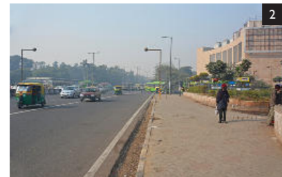
2 Pedestrian walkway along traffic island, Lala Hardev Sahai Marg
